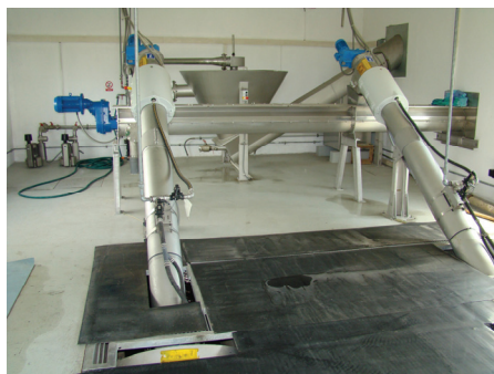
Slika 2. Rešetke i klasirer pijeska Fig. 2. Bar screens and device for sand removal
