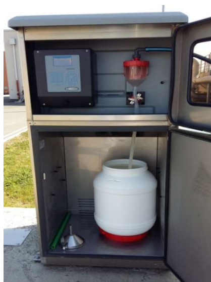
Slika 9. Automatski uzorkivač (Hach Lange) za uzorkovanje otpadne vode na ulazu u UPOV Fig. 9. Automatic sampler (Hach Lange) for wastewater sampling at the entrance to wastewater treatment plant
