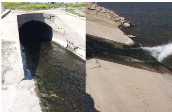
Slika 8. Izlaz pročišćene otpadne vode iz kanala u recipijent, rijeku Savu Fig. 8. Exit of purified wastewater from the canal to the recipient, the Sava river
